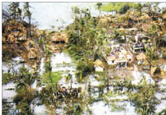
Destruction caused by a cyclone
